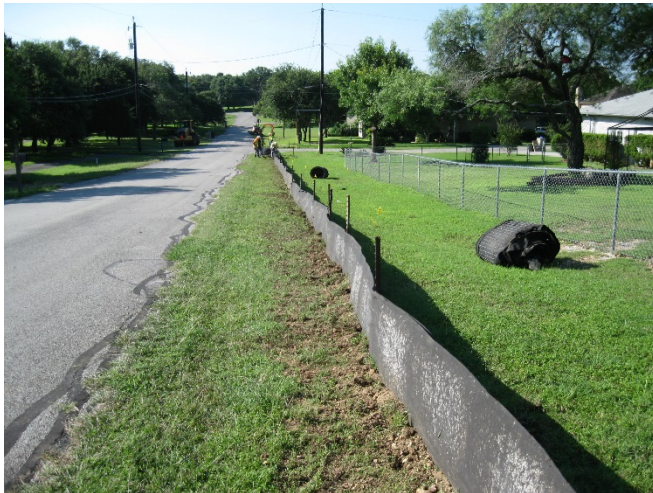
Silt fencing installed along Osage
